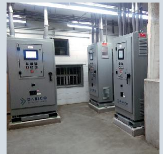
400 Hz Centralized MGs
